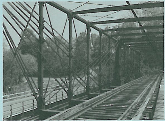
Photo 12. Baltimore and Ohio Railroad Crossing over the Little Patuxent River, Savage, Md. Two-span pin-connected Bollman through truss, 1869.
