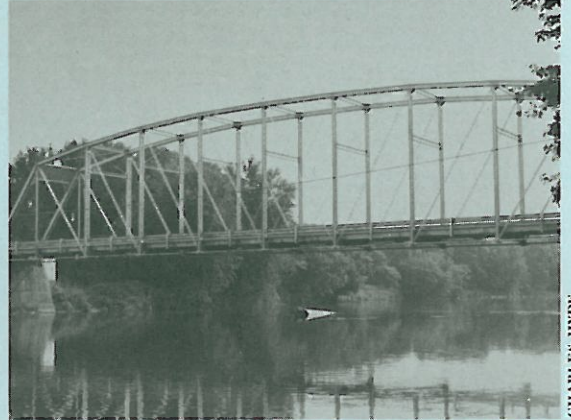
Photo 4. Portland and Danby Bridge over the Grand River, South Portlandsville, Mich. Single-span pin-connected Parker through truss, 1907.
