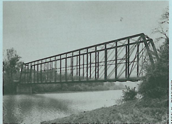
Photo 8. Laughery Creek Bridge near Aurora, Ind. Single-span pin-connected triple intersection Pratt through truss, 1878.
