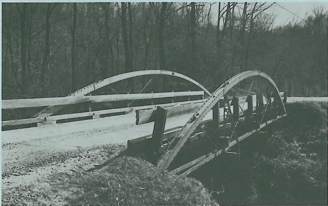
Photo 2. Roaring Run Bridge in Bedford, Va. Single-span pony bowstring arch-truss, 1875.
