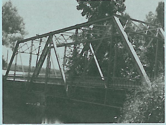
Photo 10. Studley Bridge over the St. Joseph's River, Sherwood, Mich. Single-span pin-connected Warren through truss, 1910.
