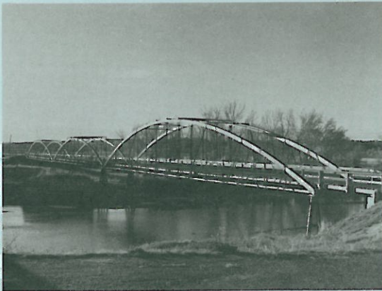
Photo 11. North Platte River Bridge, Fort Laramie, Wyo. Three-span bowstring arch-truss, 1875.
