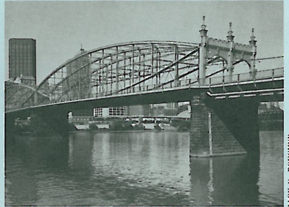
Photo 6. Smithfield Street Bridge over the Monongahela River, Pittsburg, Pa. Two-span pin-connected lenticular through truss, 1883.
